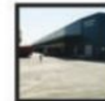
WAREHOUSE AJMER ROAD YEAR: 2021
